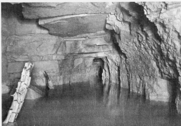
South side of the railway line. The shaft is just to the right accessible through a small hole. Remains of original timber roof supports can be seen. Photo by Nick Catford
